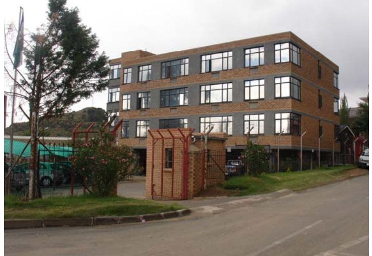
Above: The LTDC head office on the corner of Parliament and Linare Roads in Maseru.
